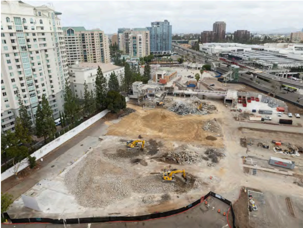
Demolition of the shuttered Costa Verde Center started in July. The developer will spend the next 12 to 18 months turning the 12.6-acre property into flat, dirt lots ready for vertical construction. The site is pictured on Sept. 16, 2026. (Luke Johnson / The San Diego Union-Tribune)
